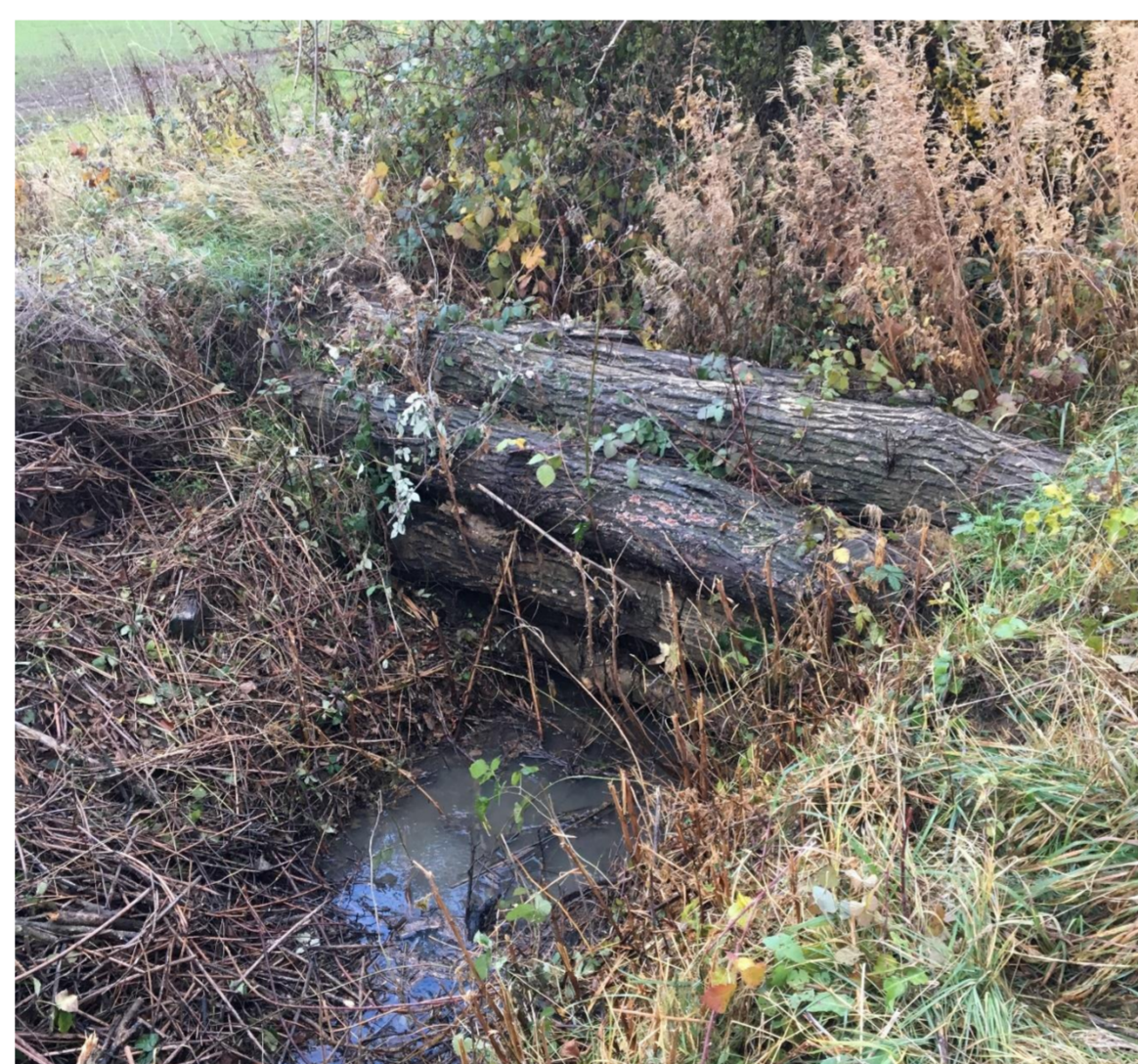
Left: Field-corner storage bunds partly filled after an intensive rainfall event in May 2018 (Image by Kestrel Photography)
