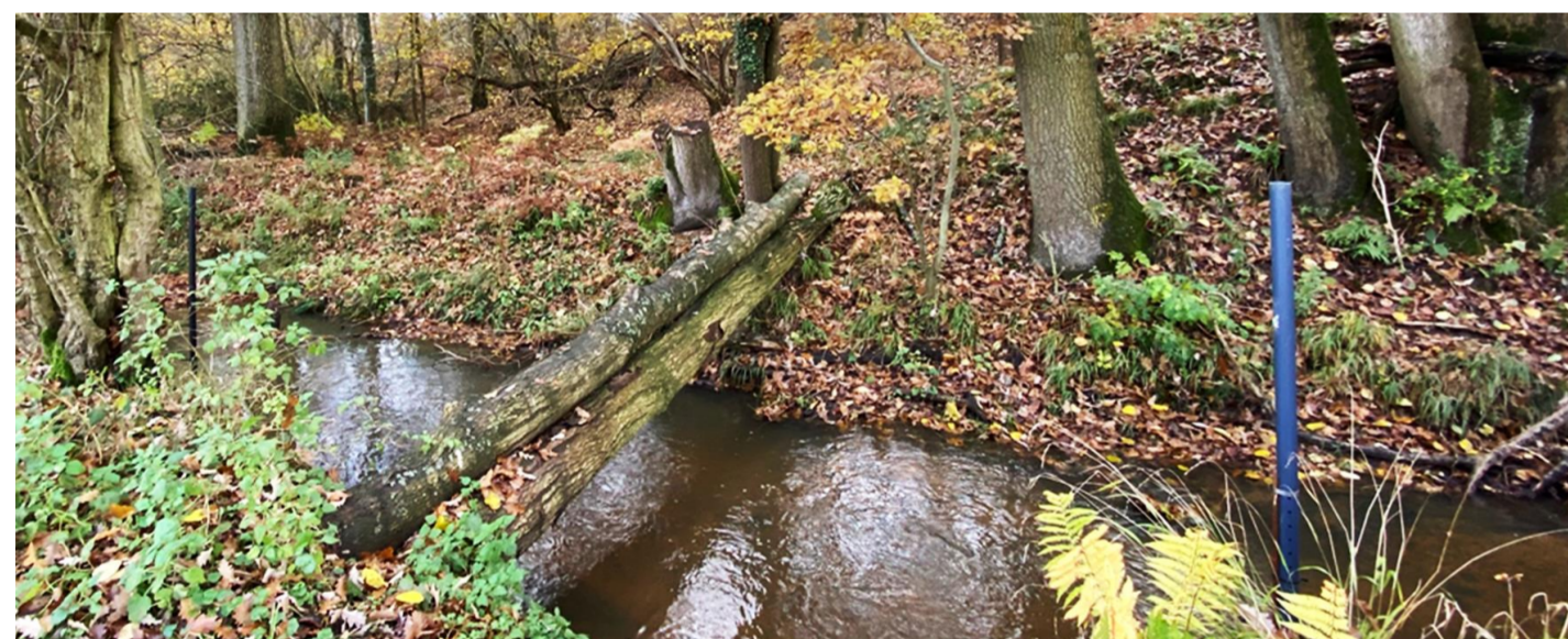
Figure 1: Pickering style leaky barrier and level monitoring equipment
