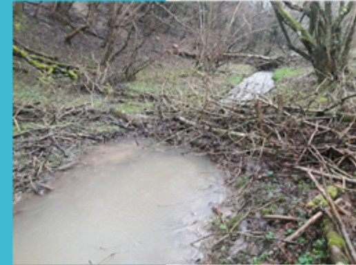
Timelapse photos of water being held back by Leaky Woody Debris Dams after high rainfall, showing how NFM can not only help slow the flow but provide additional habitat for wildlife.
