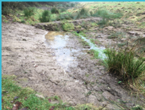
Photo of Soil Bunds holding back water. The aim of these are to intercept the water and store it temporarily, to reduce the impact of high rainfall downstream.
