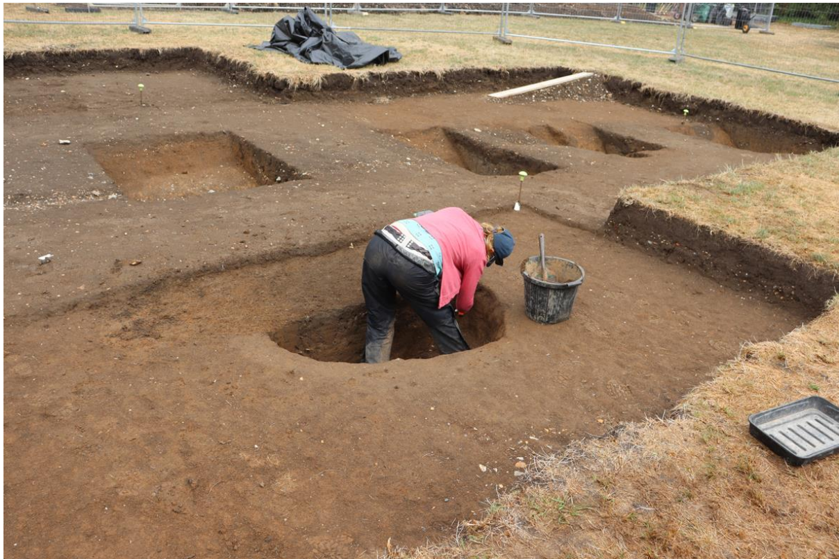
Figure 14. Pit C2304 under excavation.
