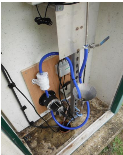
Sensor installation at a public water supply site, UK Fluorescence sensor
