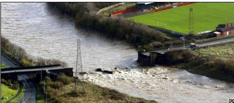
Fig. 1: Bridge collapse due to hydraulic action.
