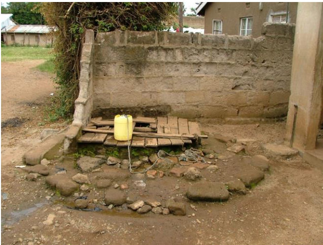
A shallow well with several potential hazards
